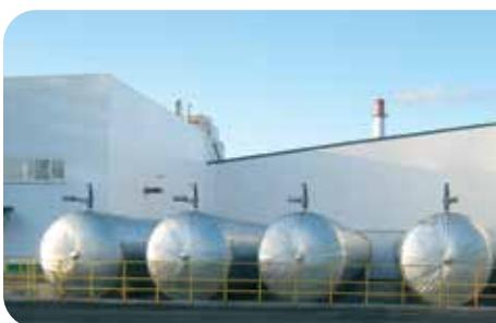
While decompressing of the autoclave the steam is used via steam distribution unit for heating of another autoclave.
